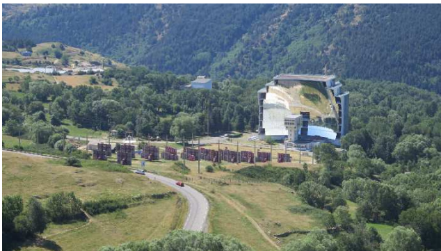
Fig. 1. PROMES laboratory at Odeillo, southern France, with the 1MW parabolic mirror. Smaller size solar furnaces are located at the southern part of the building.
